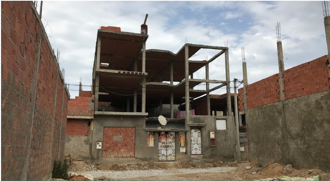
House under construction in Tunisian neighborhood undergoing ARRUs upgrading program
