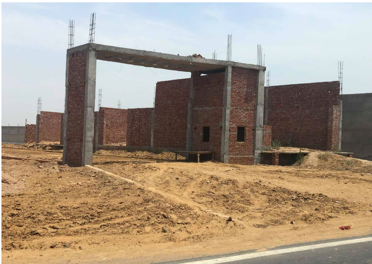
FIGURE 4. Surveillance medical officers (SMOs) would often vaccinate children of laborers clustered around construction sites
