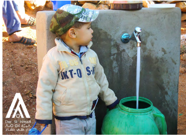
Figure 4. Water taps installed by Dar Si Hmad in villages, providing access to potable fog water
