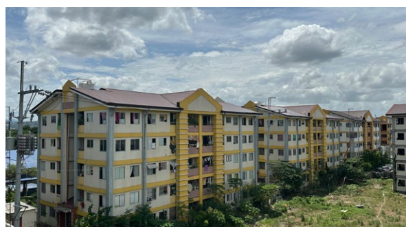
Figure 6. The Manggahan Low-Rise Building Project (LRBP) as seen from the neighbouring NHA office
