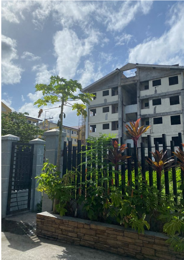
Figure 11. One of three unfinished buildings in the LRBP complex
