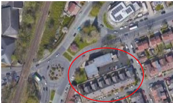
Figure 3. Aerial view of the surroundings of the temporary accommodation (circled in red), next to a busy multi-lane roundabout as well as an additional intersection in front with no zebra crossing (crosswalk) on either side
