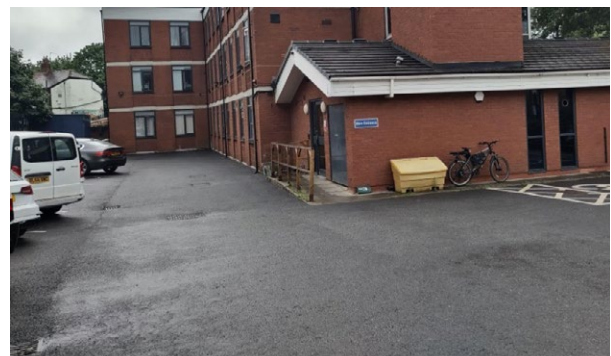
Figure 6. Exterior of TA block, Manchester
