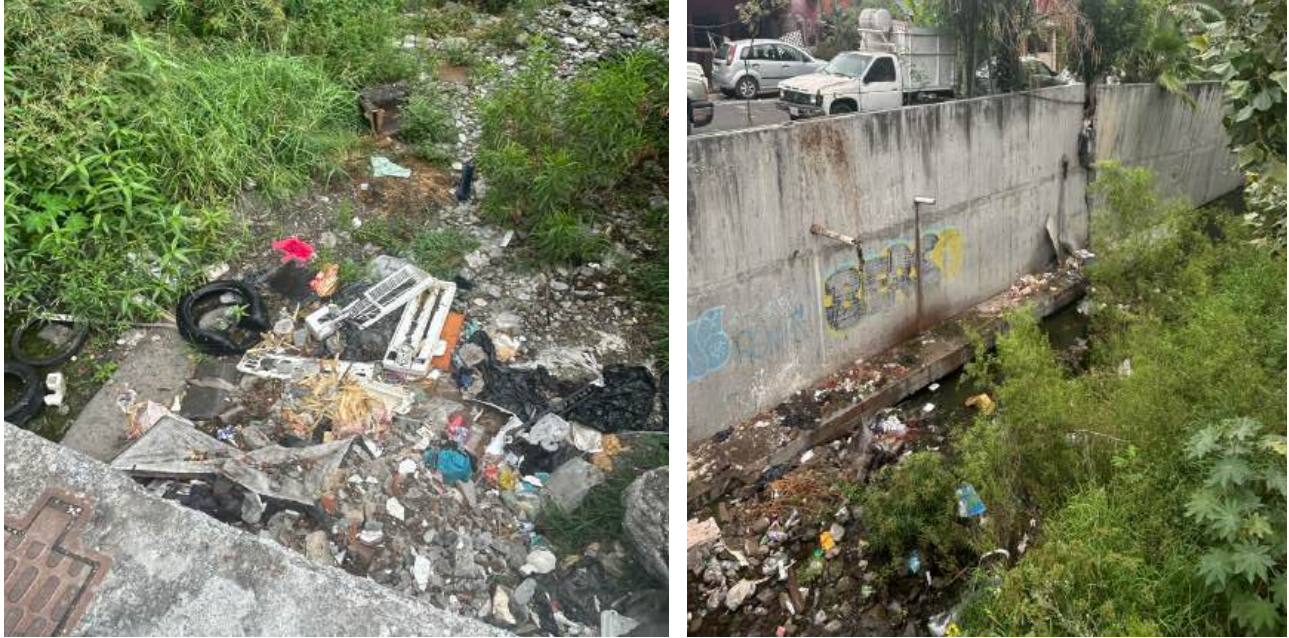
Figure 2. Arroyo Seco's current deteriorated state
